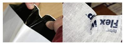
7. Form Recessed Window Corner. Remove narrow-width release paper and, using the creases made in Step 6, carefully press together the exposed butyl within the corner fold to create Recessed Window Corner. Repeat with the 3 remaining 12" pieces of **DuPont™ FlexWrap™**.
