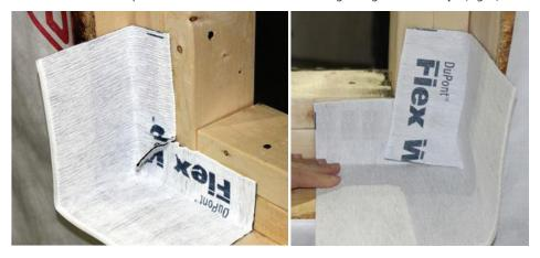
The pictures below show the 6" **FlexWrap**™ Recessed Window Corner installed on a single stud window. Note that the **FlexWrap**™ Recessed Window Corner extending slightly beyond the face of the stud (left) can be fully adhered into framing (right). See Step 4 for additional information.
