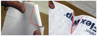
6. Crease Center Fold. Press firmly to create sharp crease in center and edges of fold. Sharp creases are necessary so the folds remain in the top sheet of the **FlexWrap**™ after release paper is removed.
